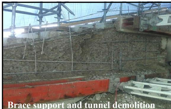
Brace support and tunnel demolition
