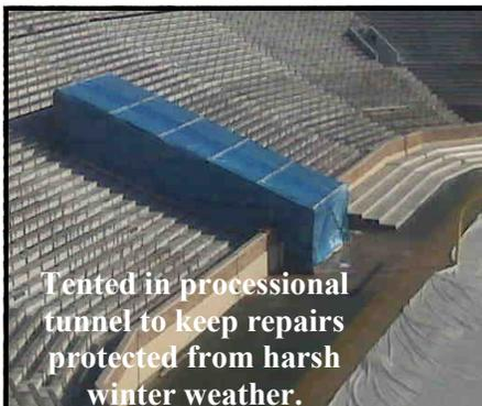
Tented in processional tunnel to keep repairs protected from harsh winter weather.
