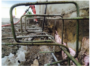
Above: concrete demolition to its bare skeleton.
