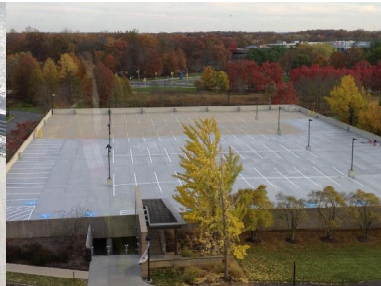
Below: Mid installation of the final traffic bearing seal-coat with the addition of anti-slip surface additives.
